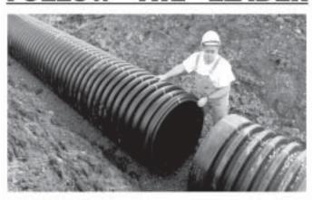
Superior customer service, experienced field engineers and knowledgeable sales representatives have earned ADS the trust of contractors and engineers for over 30 years. ADS offers a complete line of pipe and fittings in diameters 3" to 60". Construction professionals have come to rely on ADS N-12® polyethylene pipe to out perform concrete pipe when it comes to ease of installation, lower cost per installed foot, and unmatched corrosion and abrasion resistance.
